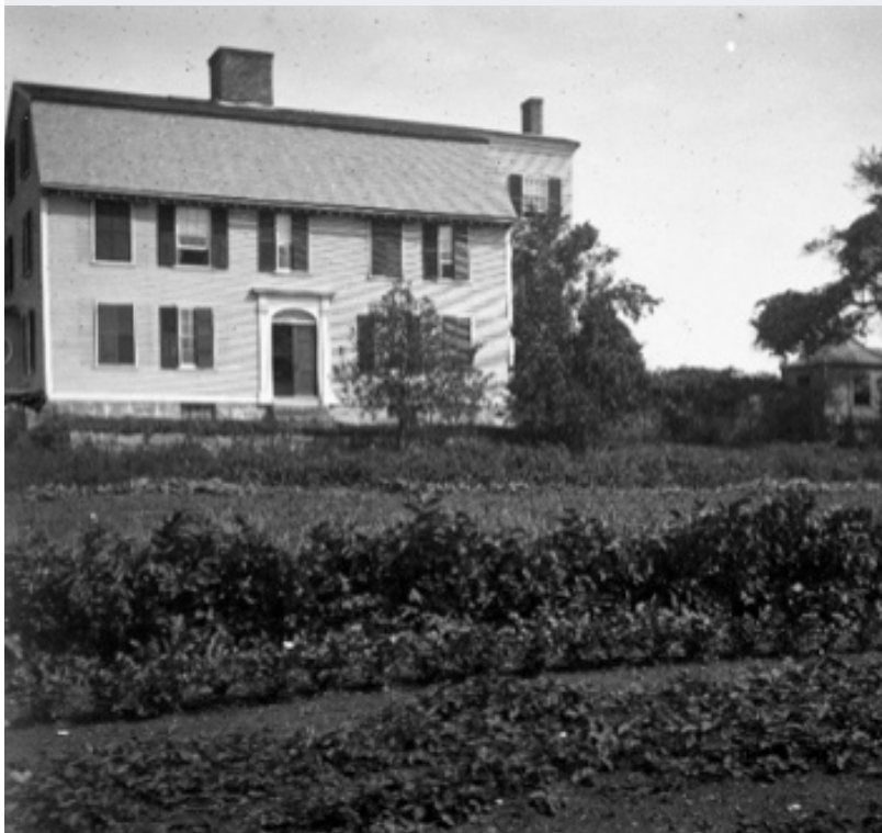
Taken in 1899, this image shows the south façade of the Babson-Alling House and the gardens which once spread out in front of it. In this photograph, the house supports a Federal-era front entryway, probably added to the structure around 1800. The property's privy (still standing) can be seen to the right of the main house.
