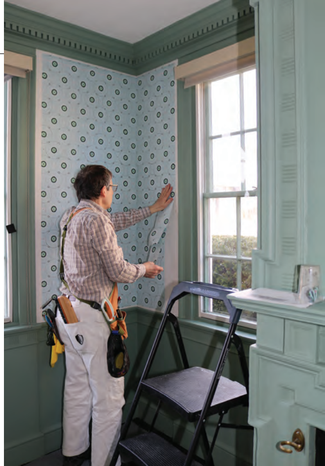
Barry Blanchard hanging the Adena Pin Ring patterned wallpaper in the front parlor of the Davis House.
