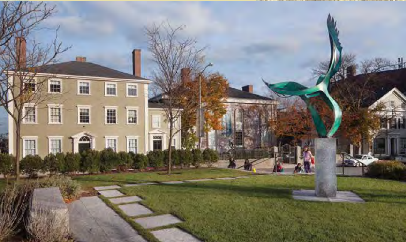
(above) View of the Museum from the park; (cover) Captain Elias Davis House, 1804, newly renovated kitchen. Photographs courtesy of Steve Rosenthal ©2014.
