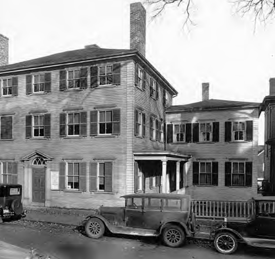
A view of the exterior of the Captain Elias Davis House (1804) as it looked when the Museum took up residency in it in the early 1920s. (Cape Ann Museum Archives)
